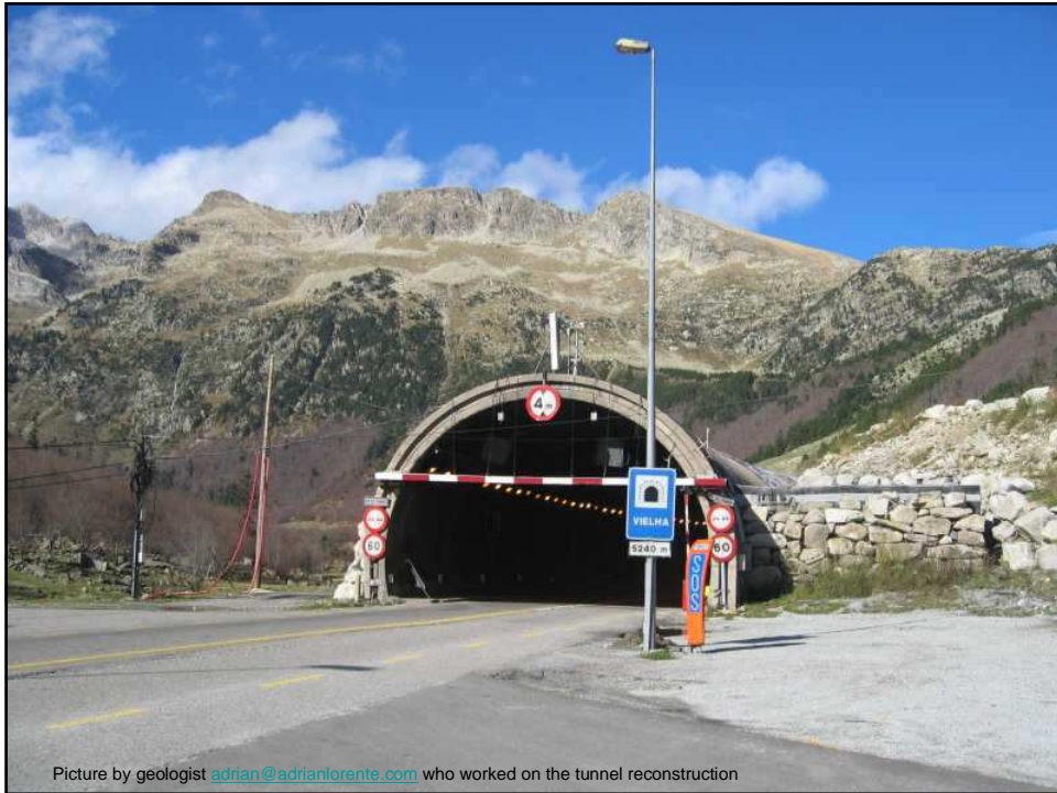
Picture by geologist adrian@adrianlorente.com who worked on the tunnel reconstruction
